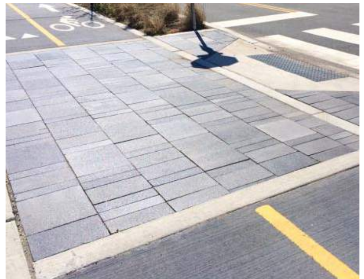
Examples of crosswalks with ornamental paving
