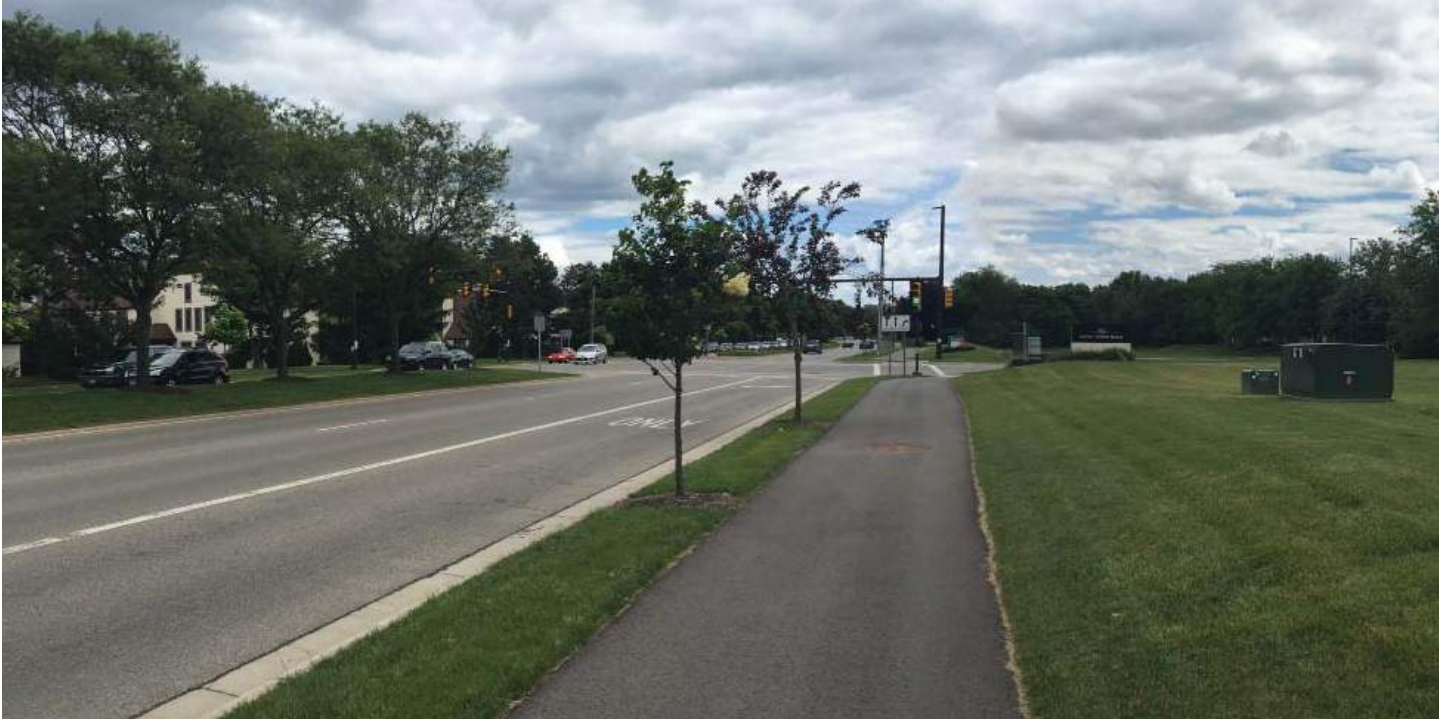
Frantz Road and Metro Place South - EXISTING
