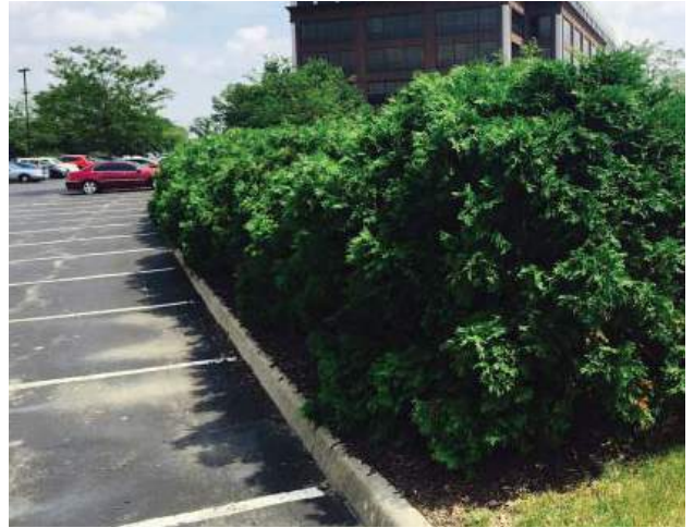
Overgrown landscaping obscuring a view of the front entrance, leading to very low usage of parking spaces.
