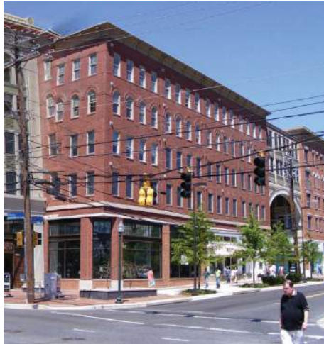
Building adjacent to the public right-of-way
