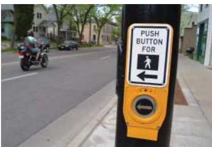
Automated pedestrian crossing signal
