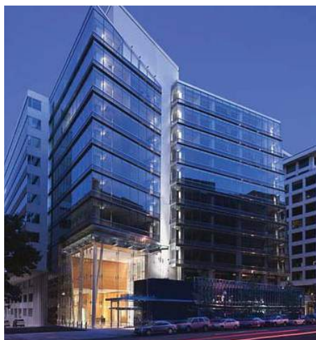
Extensive use of glass as exterior material
