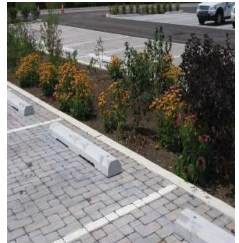
Permeable pavers in parking area
