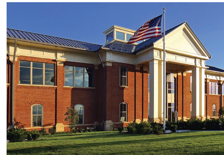
In its LEED certified headquarters, Delta Energy is a leading international provider of custom energy management consulting services for high volume energy consumers. Delta is the largest independent energy management consultant in North America and provides services to several of the largest manufacturers headquartered in central Ohio.
