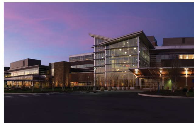
Dublin Methodist Hospital
