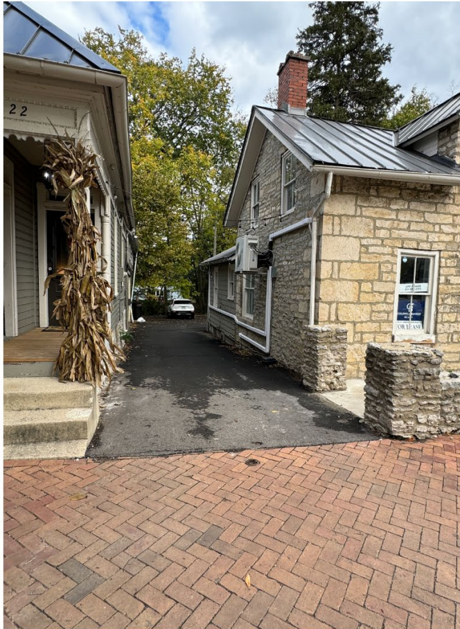
EXISTING ASPHALT DRIVE N HIGH TO REAR LOT ACCESS
